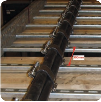
Before short circuit test
